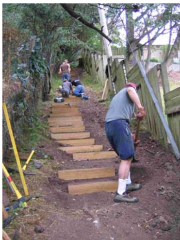
New Cedar Street path under construction
